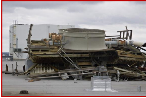
Cooling towers collapsed by high winds
