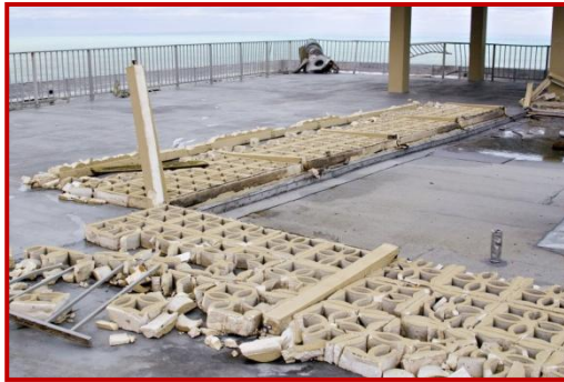
Roof observation railings collapsed
